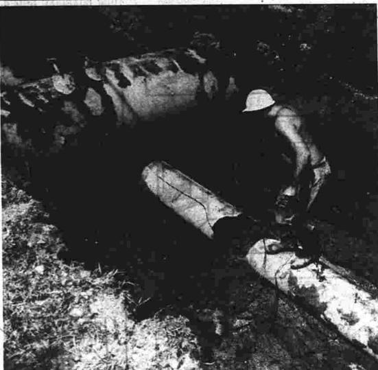
The split in this water main is why so many households in the northwest corner of Vernon were without water today. The gaping hole in the main was cut by workmen to ease removal of the cracked section. The larger pipe is a State Highway Department storm drain whose weight finally cracked the water line. Workmen at the scene this morning noted there were no concrete
